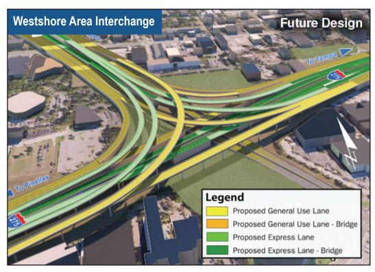
Local street improvements to enhance mobility would include the reconnection of Reo Street, Occident Street, and Trask Street under I-275 providing additional north-south connectivity. A new on-ramp from Reo Street to southbound I-275 would provide direct express lane access. A diverging diamond interchange at Reo Street will provide new connections between Kennedy Boulevard and Cypress Street.
